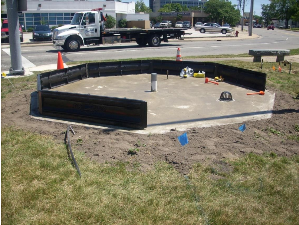
Image 06: Example of walls being laid out for Root Park Fountain
