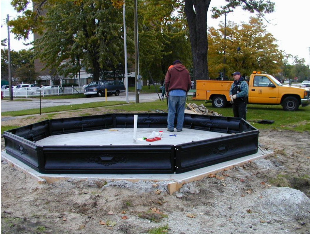
Image 08: Example of the walls in place for Kearny Park Fountain
